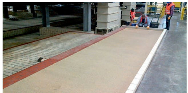
Installing a screed coating
