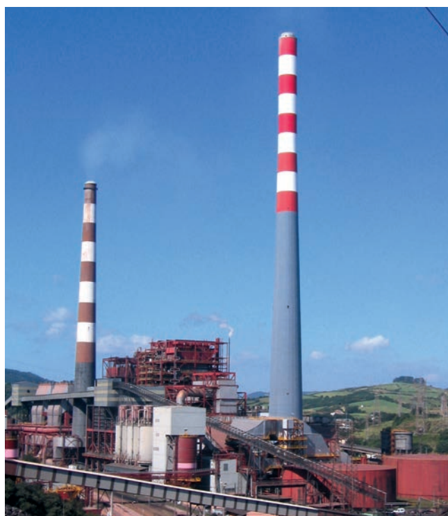
Coated power station chimney
