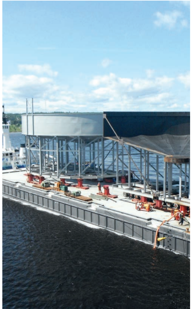
Delivery of rubber-lined thickener parts
