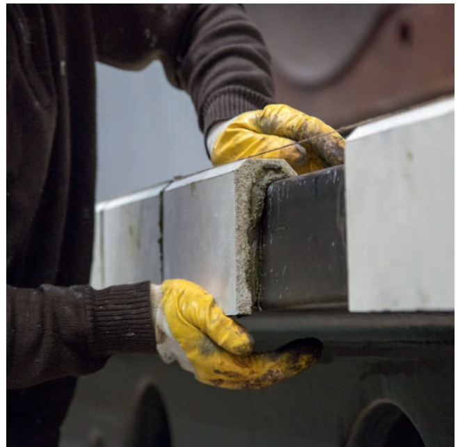
Working with synthetic resin mortar
