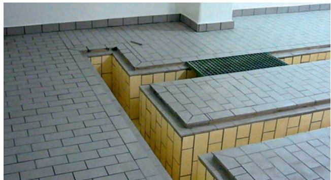
Combined covering implemented with gutters
