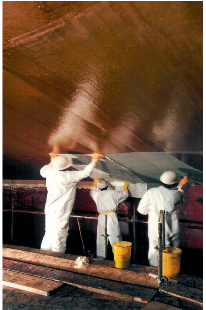
Installing a laminate coating
