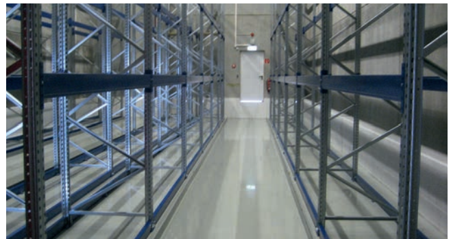
WHG coating in a shelf storage warehouse
